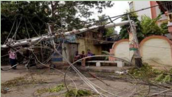
Hanging electric pole (The Hindu)
